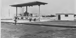
The new main facilities where jet fuel, gasoil, motor gasolines and aviation gasoline can be loaded safely and efficiently can be seen here with a small office for the loading rack operator.
